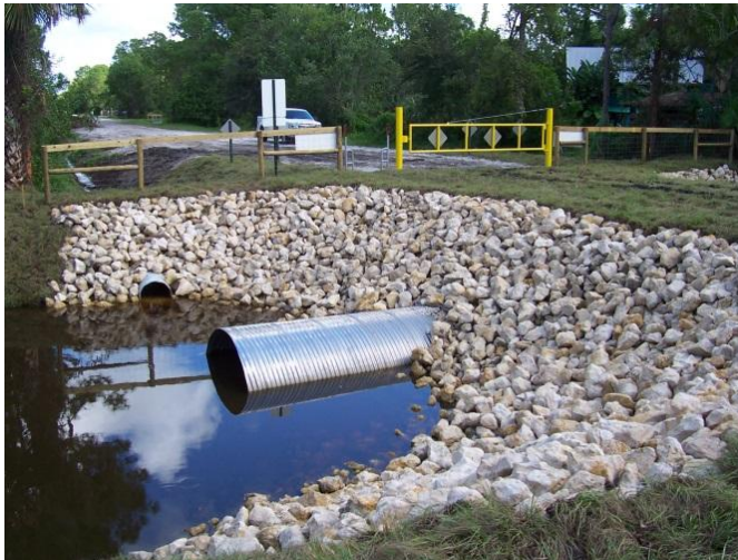
Figure 8. Canal 7 Culvert at Alexander Run
