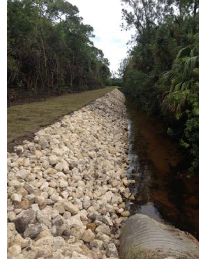
Figure 7. Canal 18 looking North
